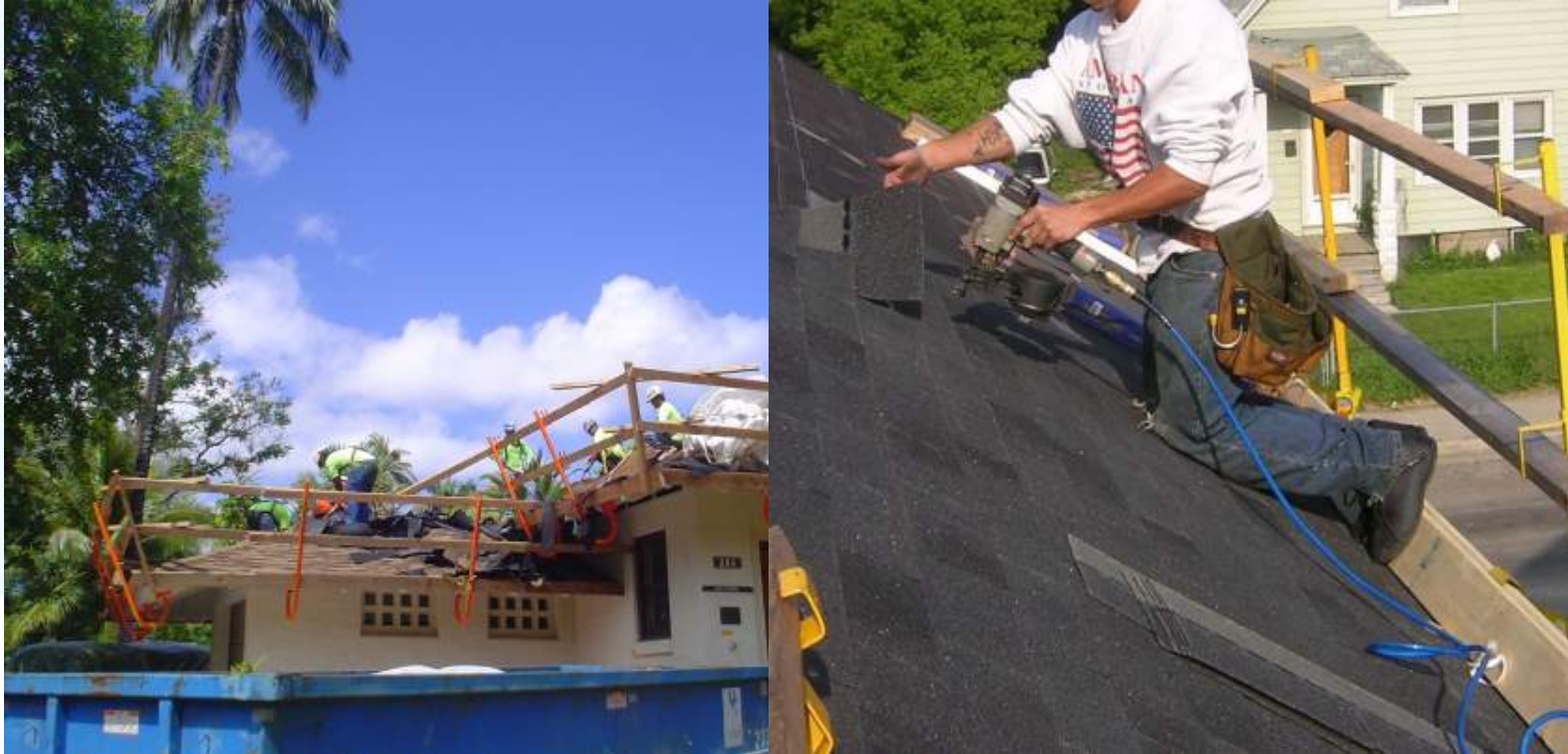
Guardrails in place during re-roofing activities.
