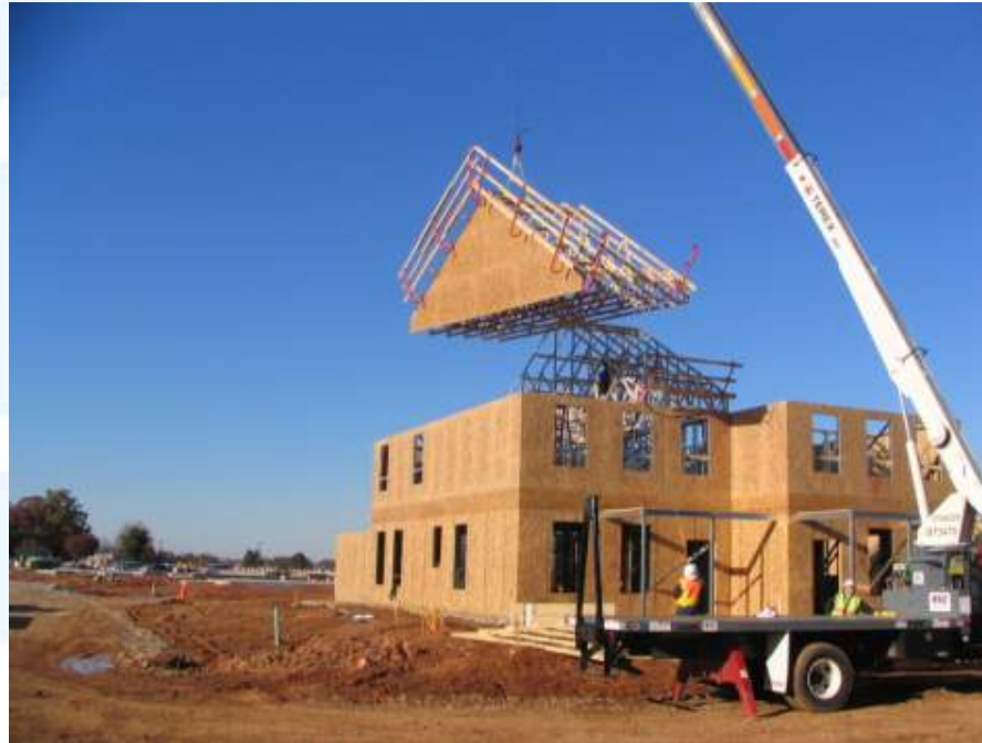
Pre-installed fall protection
